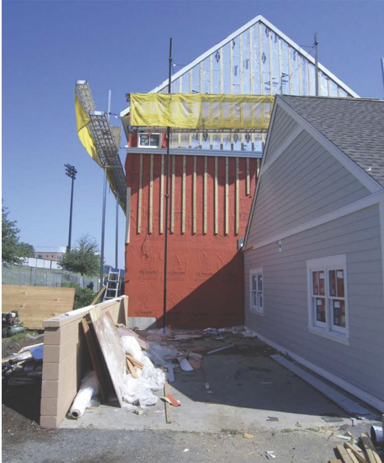
A retrofitted wall complete with ENERGY STAR-rated, aluminum-clad, double-hung wood windows stands next to an under-construction wall showing the orange air barrier and blue non-structural rigid insulation.
