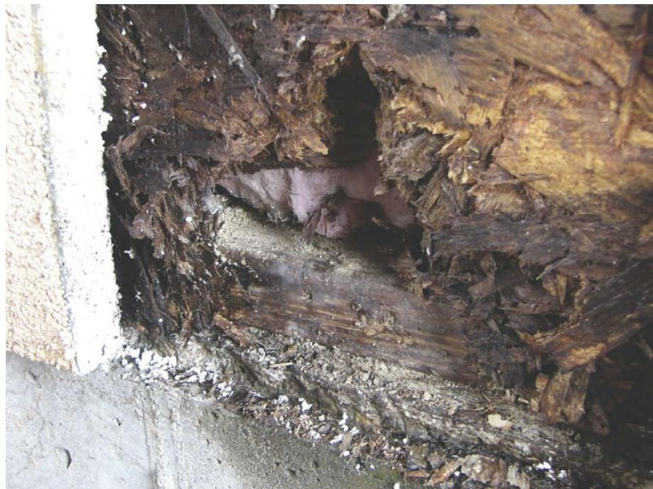
Test cuts reveal unadhered EIFS and deteriorated sheathing and sill plates.
