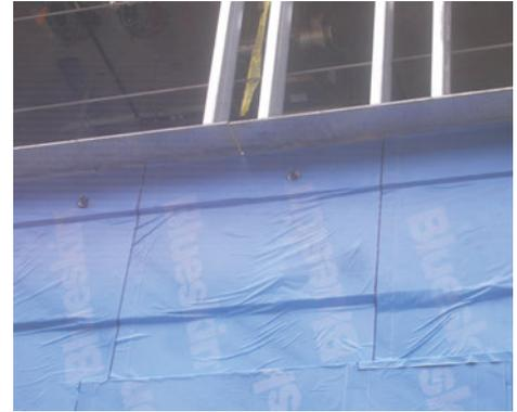
*The air barrier membrane is wrinkled, tented over projections in the substrate and spanning over substrate changes in plane at the North Carolina science building.*
